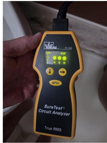
27 120 VAC shore-power polarity verified correct (circuit analyzer).
