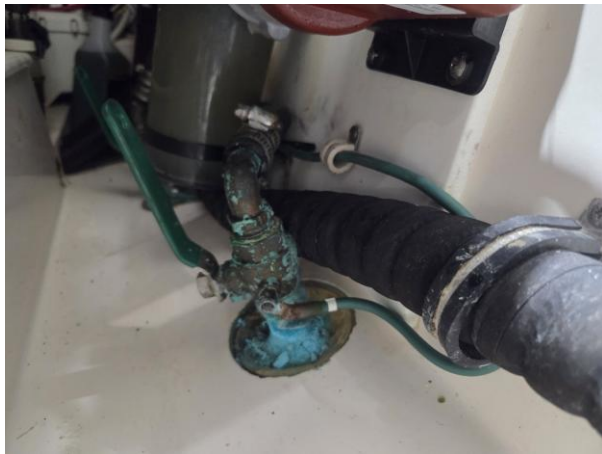
28 Bonding established to metallic thru-hull fittings; no galvanic or electrolytic corrosion sighted.
