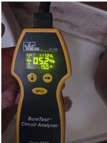
38 Generator tested satisfactory under load.
