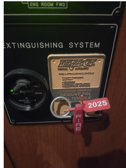
82 Manual fire suppression controls at the flybridge and pilothouse helms
