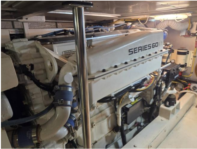
19 Detroit Diesel Series 60 main engines
