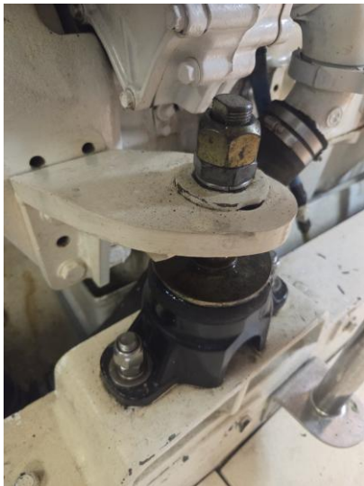
25 All engine mounts clean and corrosion-free
