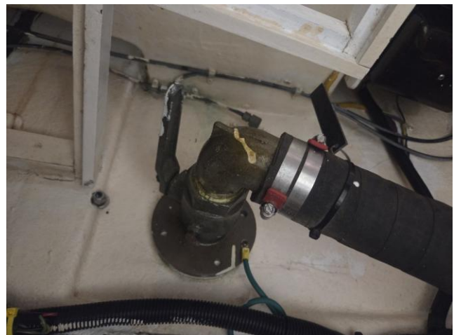
68 Seacocks operated; thru-hull bonding clean, corrosion-free and well terminated
