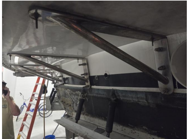
12 Swim platform well secured; no significant corrosion at brackets or fasteners
