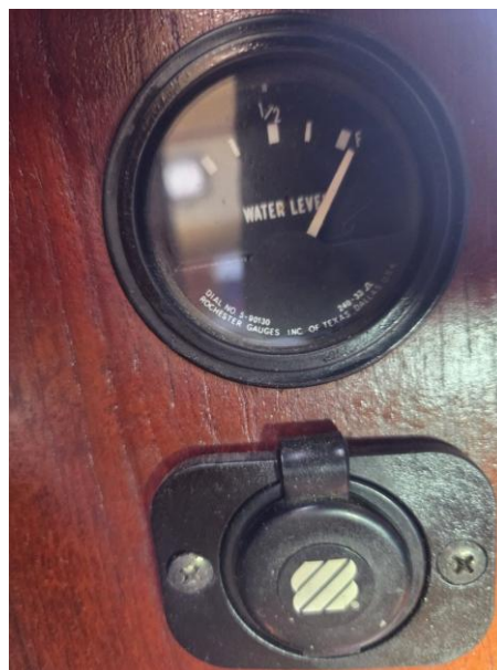
60 DEF Water tank gauge is not correct
