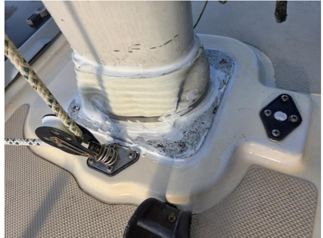
13 Mast partner well sealed; no leaks observed from the interior
