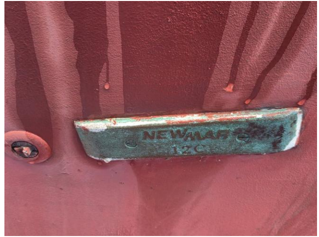
11 Bonding ground plate clean
