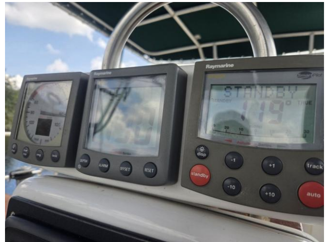
52 DEF All instruments power up; wind direction and speed transducers not mounted on the mast
