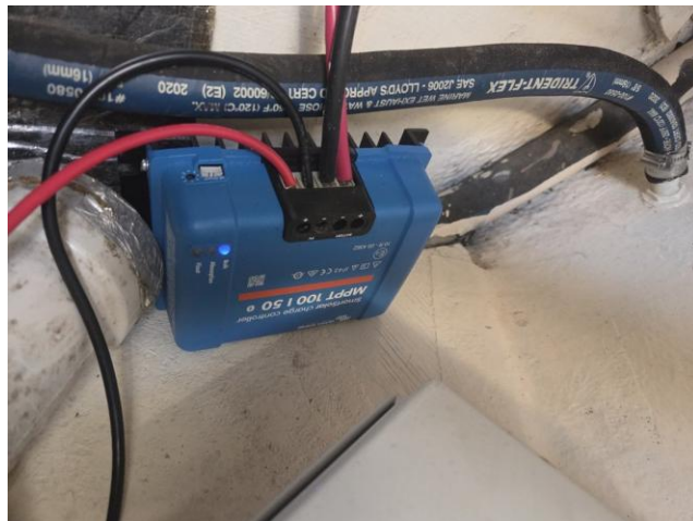
48 Victron SmartSolar MPPT controller operating as intended
